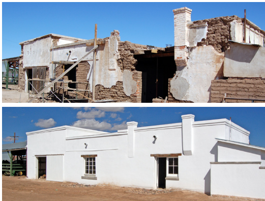
Top – Headquarters buildings under repair. Bottom – Headquarters buildings rehabilitated. Photos by Simon Herbert
