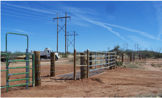
New Empirita fencing and gate for access control. Photo by Joe Kellner
