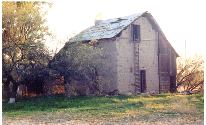
Southeast corner of Pump house. Date unknown. Courtesy Arizona Historical Society
