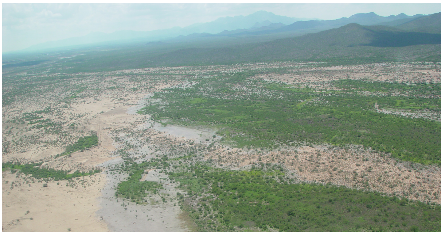
Flooding in 2005 along the Brawley Wash north of the Bee & Mordka properties, looking northeast across the Tucson Mountains. Photo from Regional Flood Control District.
