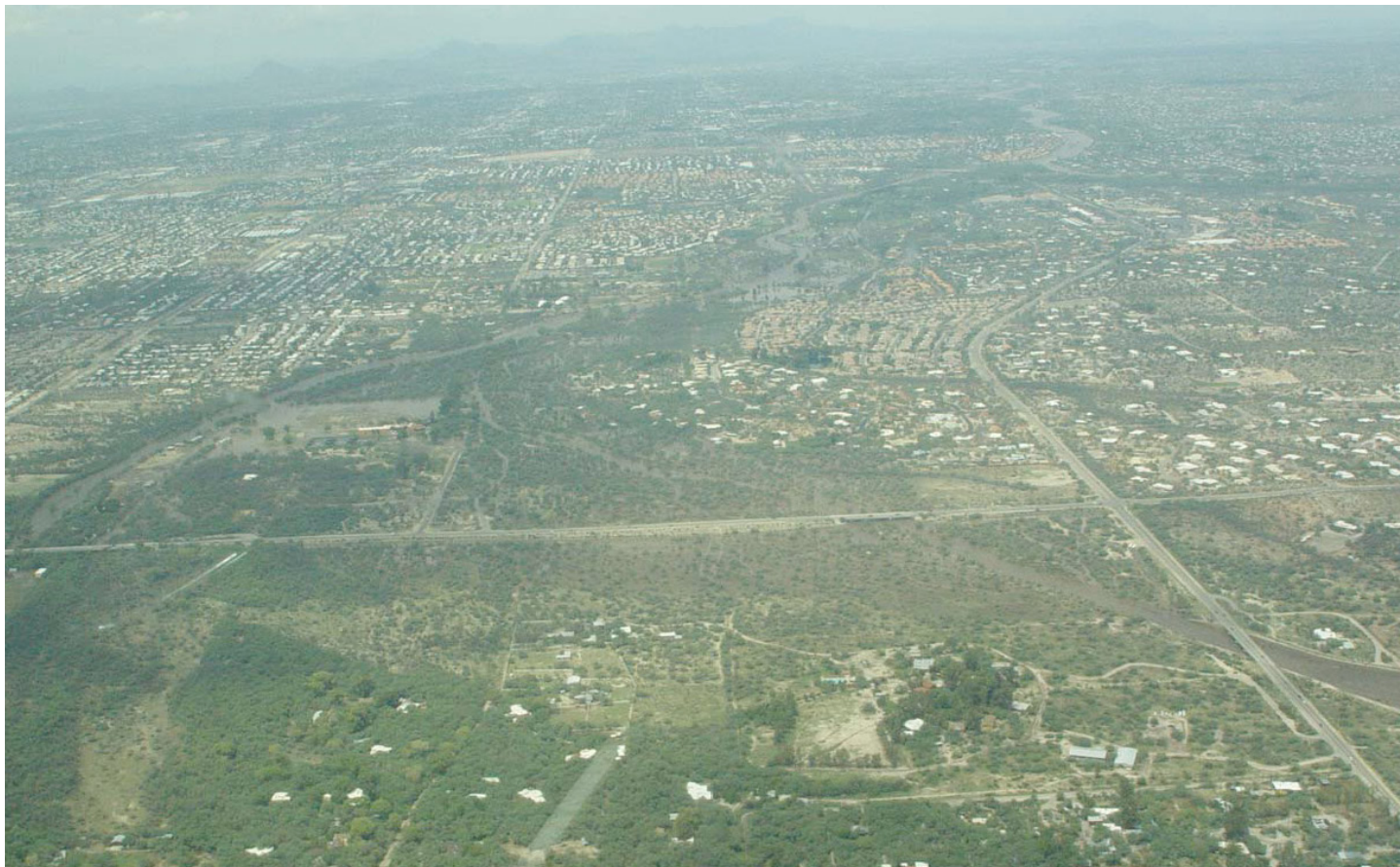
Looking west at the confluence of the Agua Caliente Wash and Tanque Verde Creek. Photo shows over bank flooding on both sides of Houghton Road, which is visible through the center of the photograph. Photo by Terry Hendricks, July 2006
