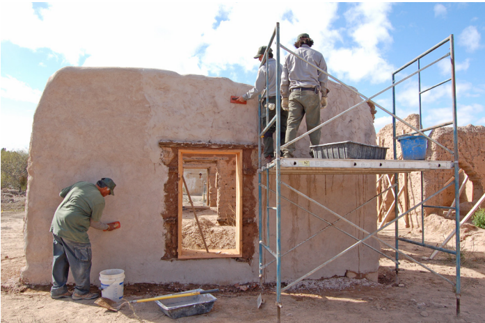
Reconstruction work at Fort Lowell - Photo by Cultural Resources Office staff.
