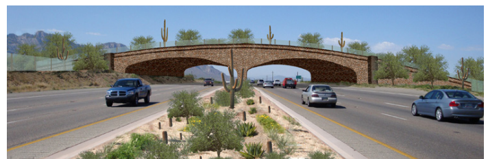
Oracle Road - street view with Overpass
