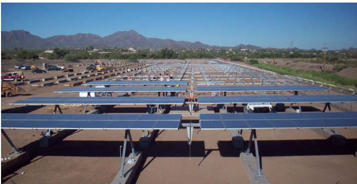
Photograph of the 1 megawatt solar generating facility at Pima County's Roger Road Wastewater Treatment Plant. The County would like to use portions of the land acquired around Davis-Monthan Air Force Base for solar generating facilities in order to increase the amount of renewable energy resources used for County operations.
