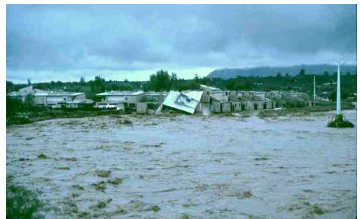
Flood damage, First Avenue and Rillito Creek 1983
