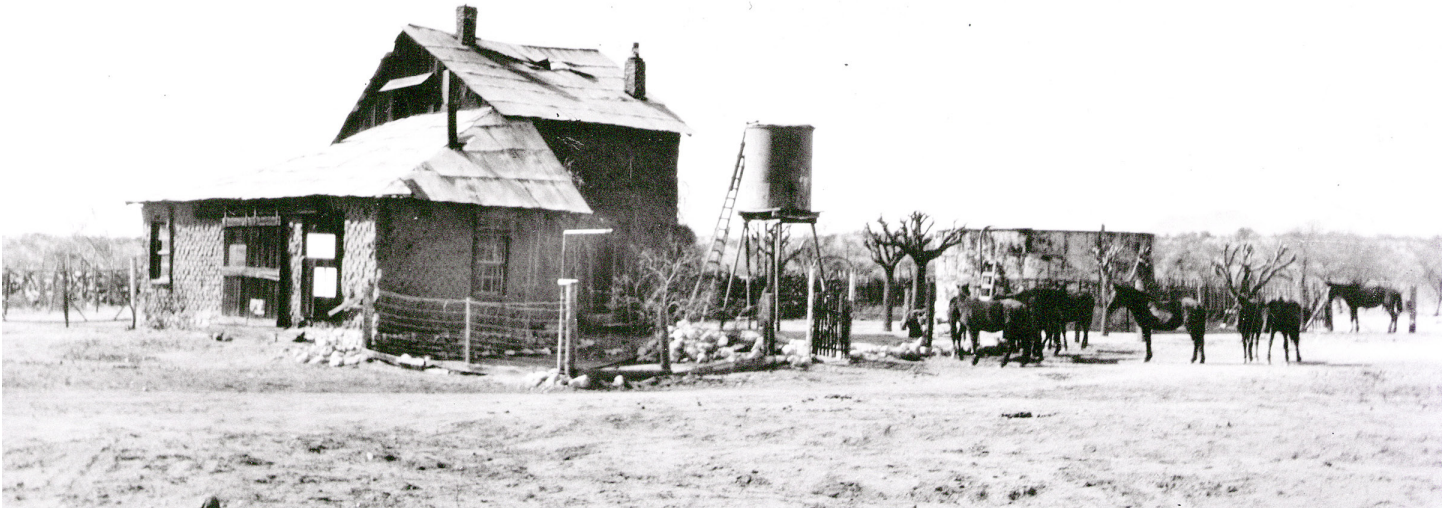
Northeast corner of Pump house ca. 1900. Courtesy Arizona Historical Society
