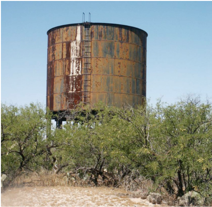
The Pantano Water Tank still stands by the Union Pacific railroad crossing through the Townsite - Photo by Cultural Resources Office staff.
