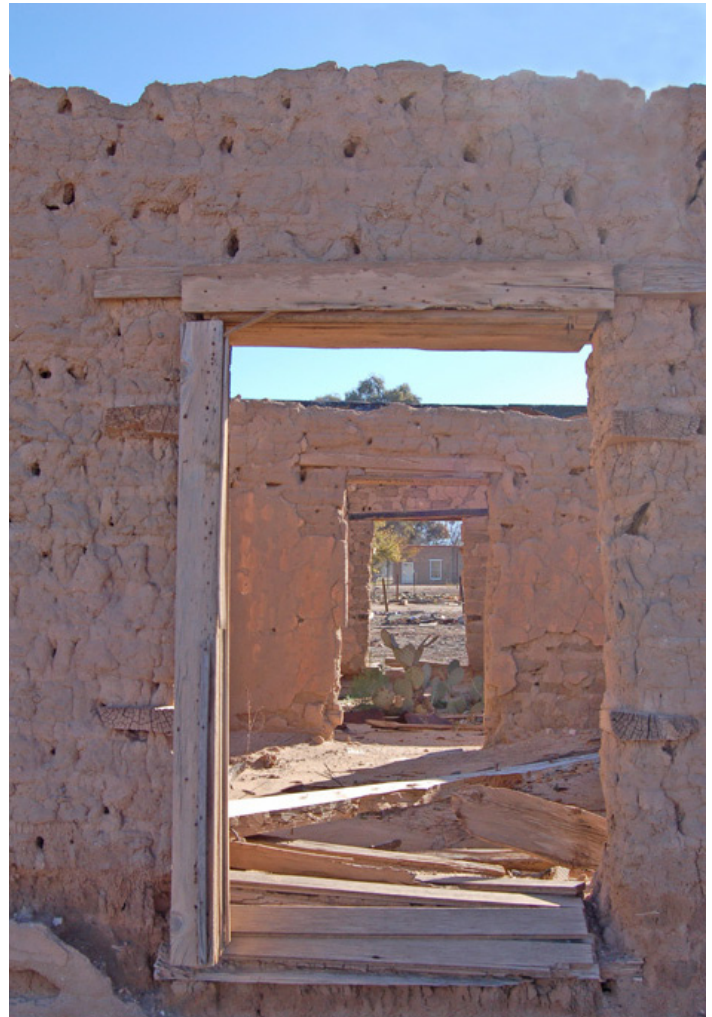
Fort Lowell adobe buildings - Photo by Cultural Resources Office staff.
