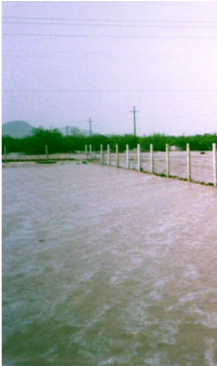
Blach Wash flooding roadways, 1990
