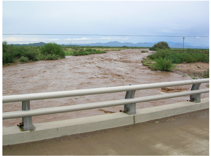
Ajo Highway bridge crossing the Brawley Wash looking north. Photo from Regional Flood Control District.
